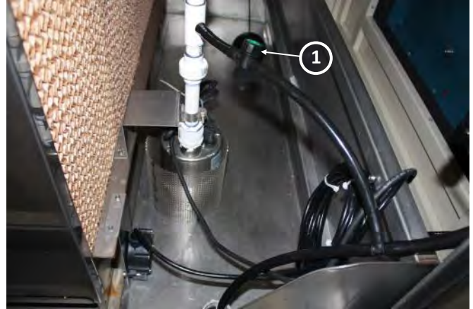
FIGURE 19- BLEED RATE ADJUSTMENT
