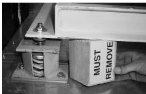
FIGURE 7 - SHIPPING RESTRAINTS
