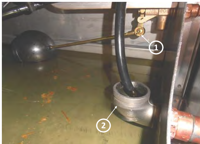
FIGURE 16- SETTING WATER LEVEL
